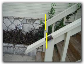
$\square$  Improper dimensions of stair raisers - steps are not recommended to be taller than 7 3/4" - noted at the bottom of the rear stone steps
