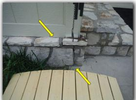
☑ Inadequate clearance between siding and grade - recommended to have 4" - 6" of clearance - noted in the rear of the garage
