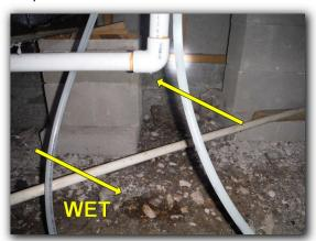
$\ensuremath{\square}$  Water pipes are not recommended to be supported with bare wire - noted below the utility room
