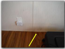
☑ Cracks in the sheet rock wall covering - noted over the rear family room exterior door and left rear window in the family room, and above the right rear bedroom door opening
