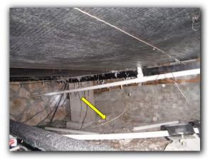
☑ One or more connections are not in junction boxes - noted above the fan in the rear garage storage room
