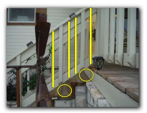
Hand railing is not terminated properly - recommended to be terminated at the last post to prevent snagging clothing or accessories and causing a fall - noted at the front porch steps
