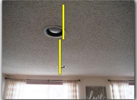
☑ Evidence of a patch or repair to the ceiling sheet rock - noted near the light fixture in the dining
