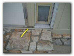
$\ensuremath{\square}$  Wood siding is soft or damaged in some areas - noted along the bottom of the rear walls of the garage
