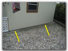
$\square$  Some cracks noted in the stone skirting material - noted in the front of the home near the hose bib and at the right outside corner of the rear porch
