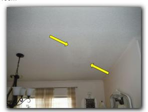
☑ Staining on the ceiling sheet rock - noted near the fan in the breakfast area
