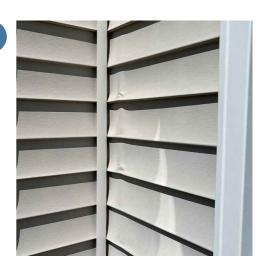
3.3.3 Wall-Covering, Flashing & Trim **HOLE IN SIDING**
