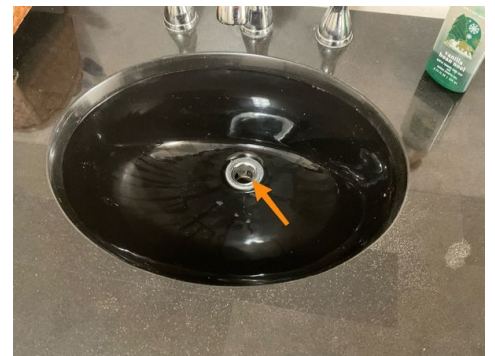
2nd Floor Bathroom
