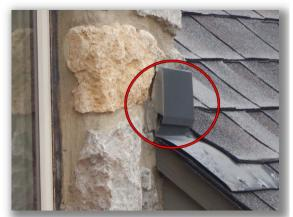
• There was no kickout flashing details observed at the lower bottom edge of the roof line interface and the sidewall that continues past the edge of the roof(various areas around the house). The lack of this kickout flashing may allow water to penetrate at these points. No significant problems were observed at time of inspection due to the absence of the kickouts.
