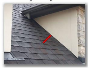
• Any missing or deteriorated sealant, observed at the flashings at the front dormers, should be replaced.
