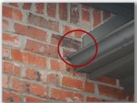
• The counter flashing should be properly installed.(observed at the front right side of the house about where the garage meets the house) This condition is typically addressed at time of next roofing or if damages occur. Until repairs are undertaken openings/gaps between the flashing and side walls should be sealed.
