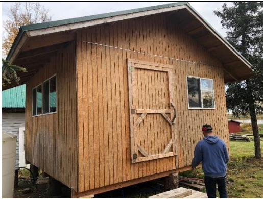
New Processing Building
