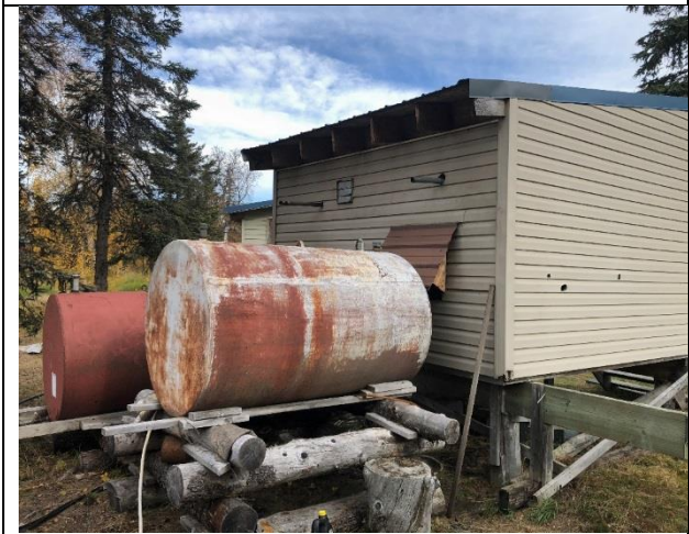
Generator Shed - Rear
