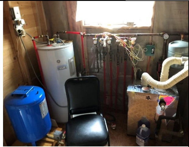
New Building / Bunkhouse - Interior
