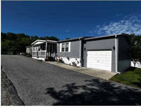
Exterior One Car Garage View
