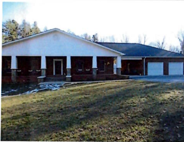
Main Structure Photo
