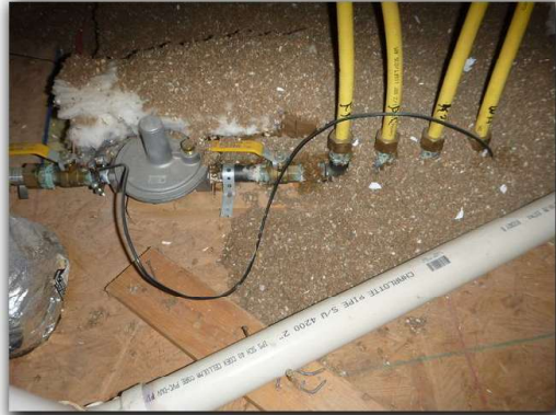
Example of proper bonding
