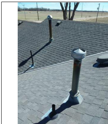
Middle of Roof North
