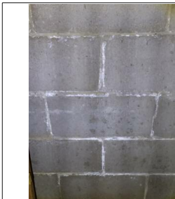
South wall East
