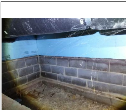
North wall East
