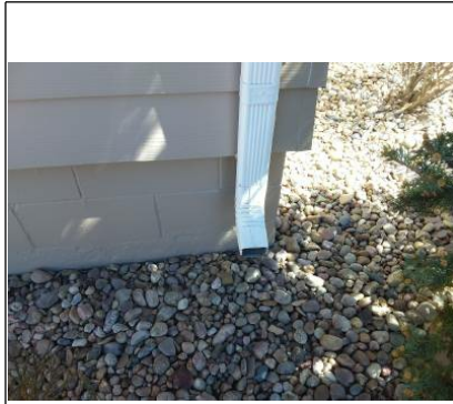
West wall South
