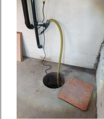
Northeast room Southeast corner
