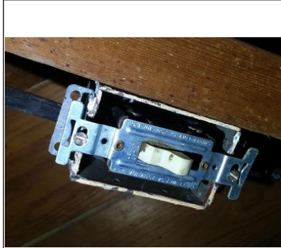
South central room Southwest ceiling
