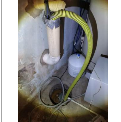
South Central room North
