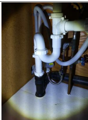
Under Kitchen sink
