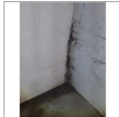
Southeast lower walls and floor
