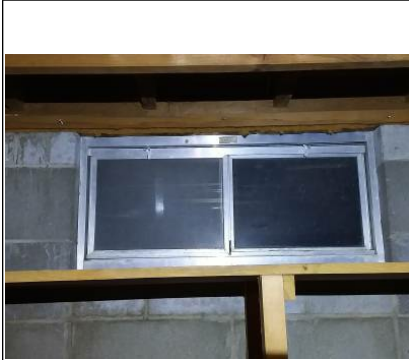
North wall East
