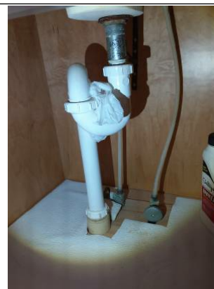
Under first floor hallway Bathroom sink
