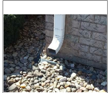
East wall South
