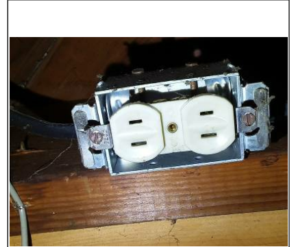
South central room East ceiling
