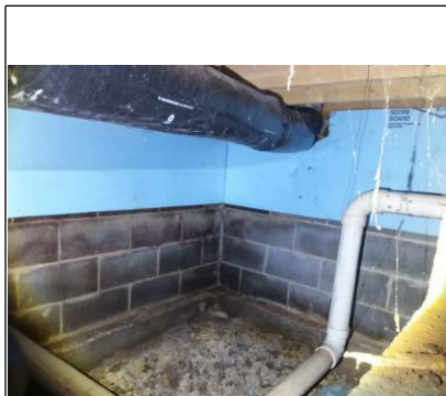
North wall East
