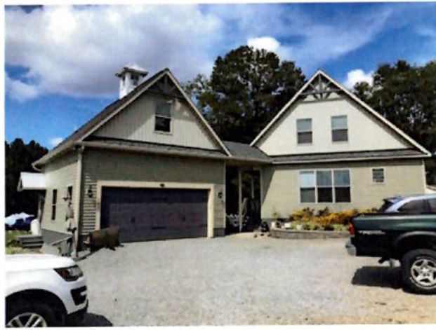
Main Structure Photo
