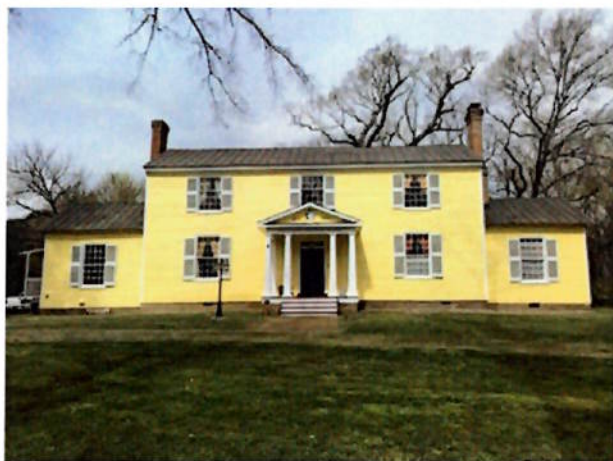
Main Structure Photo
