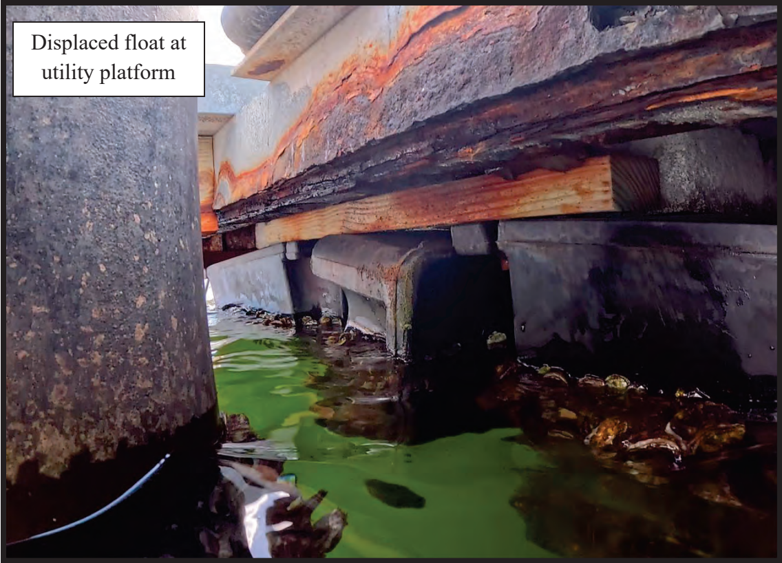
Heavy utilities deflecting wooden brace
