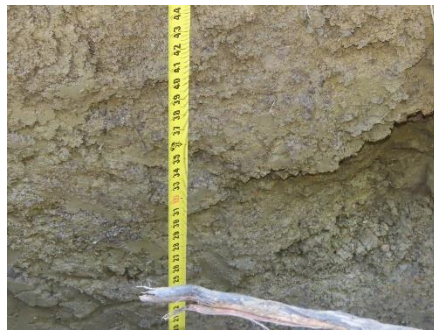
Figure 2 – Wall of Deep Test Pit Hole
