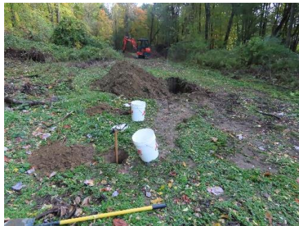
Figure 3 – Perc Test Holes
